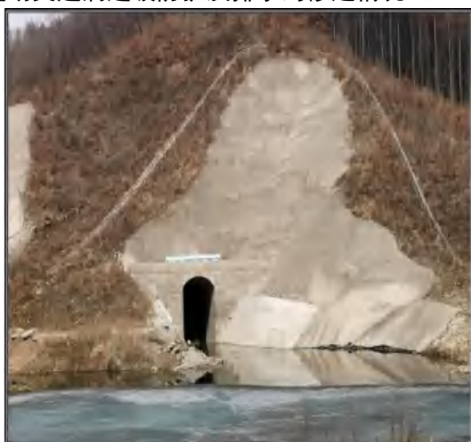
排水洞洞口边坡防护情况 (2021. 3)
