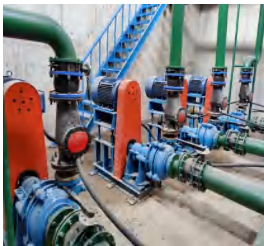
浓缩池渣浆泵
